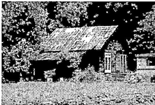
Phillip Lowe House
