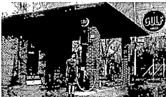
Blake's Brick Station
